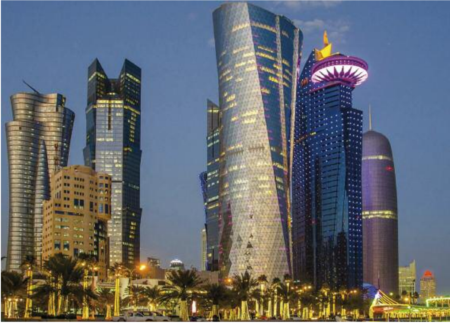
Noc Tower, Qibla Qatar International Islamic Bank _ Doha _ Qatar
